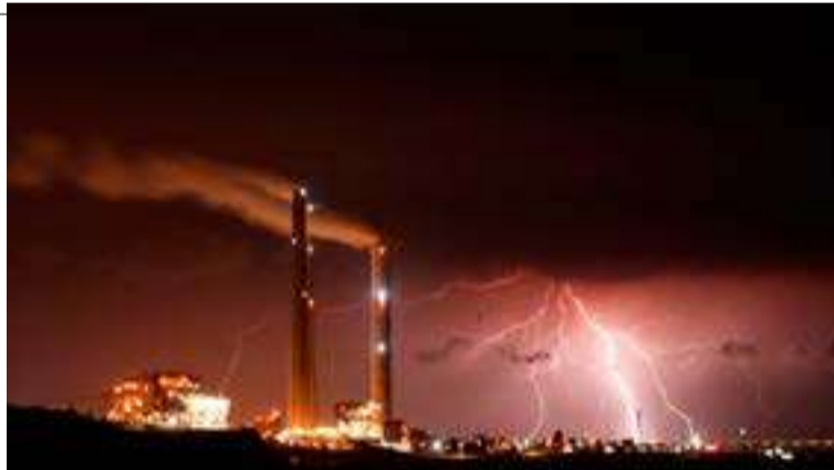
Rutenberg power station is seen as lightning strikes over the Mediterranean sea at the coastal city of Ashkelon, Israel. REUTERS/Amir Cohen
