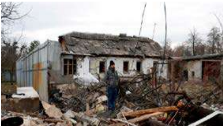
A man stands at a site of a residential house damaged during a Russian missile strike in Kyiv, Ukraine December 29, 2022. REUTERS/Valentyn Ogirenko
