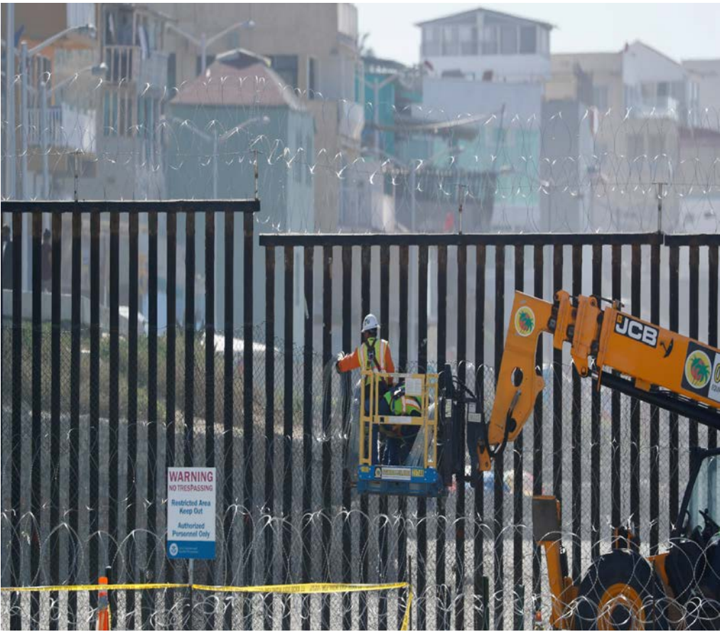
Workers on the U.S. side install concertina wire along the border fence between Mexico and the United States at Border State Park in San Diego, California
